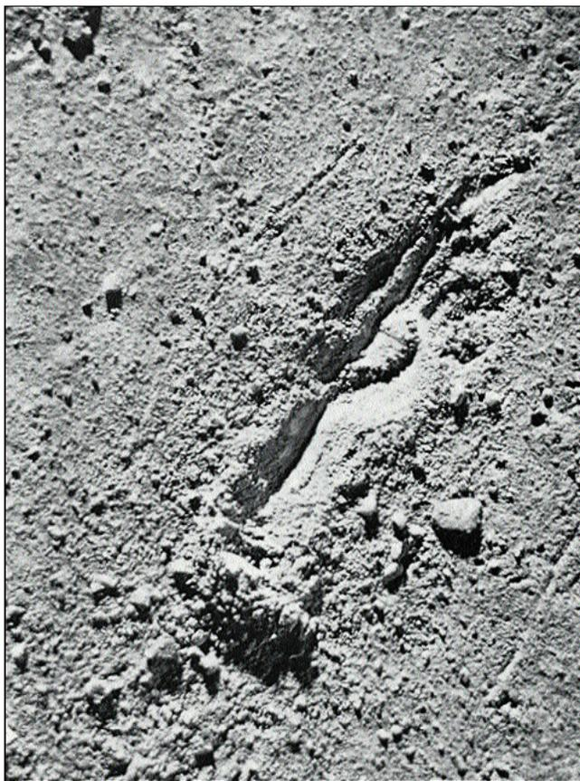
Close-up view of a severely dusted concrete floor slab scratched with a sharp instrument.
